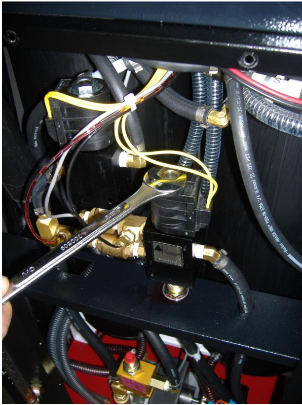
2. Take off nut with a \frac{3}{4} " wrench. To remove coil pack
